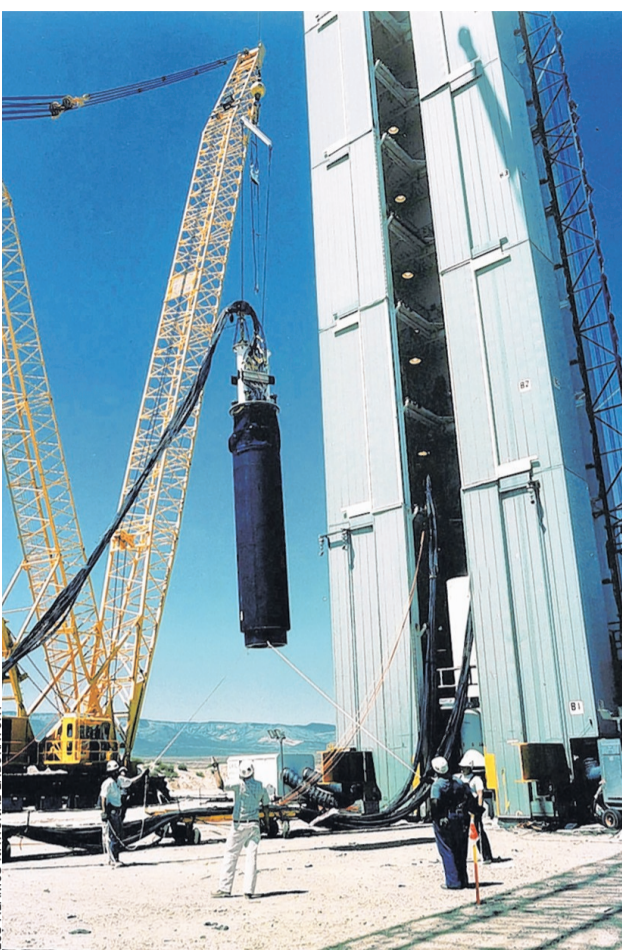
Hoisting the rack for the U.S.'s last full-scale nuclear test, 1992.
